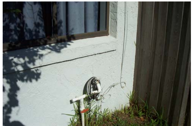
Siding has moisture damage, needs to be repaired. Connection to irrigation system is health hazard.
