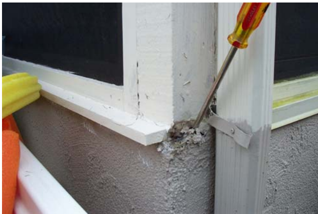
Siding has moisture damage, needs to be repaired. Connection to irrigation system is health hazard.
