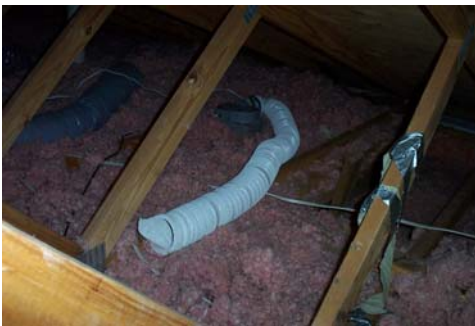
Exhaust vent in attic
